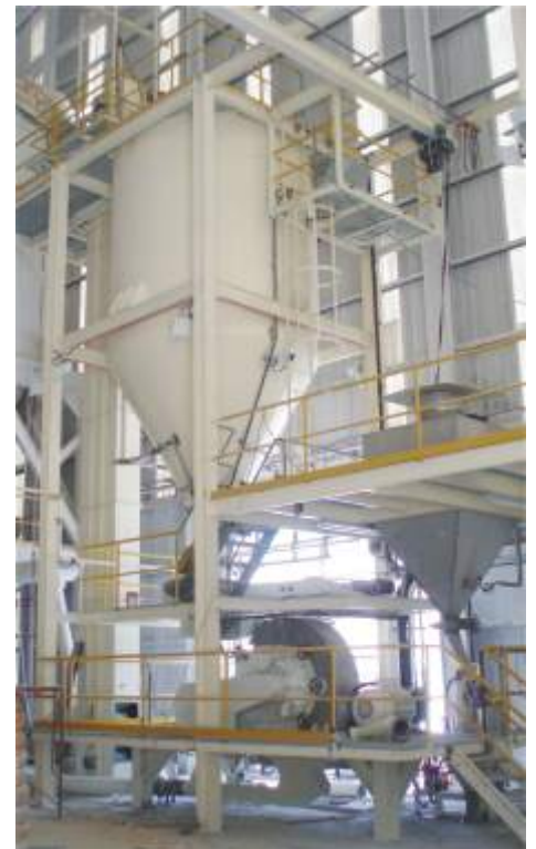
2. SMW 63 in a coating installation
