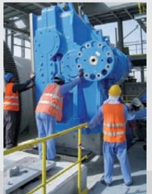
Traditional pinion/gear rim drive with grease spray lubrication.
