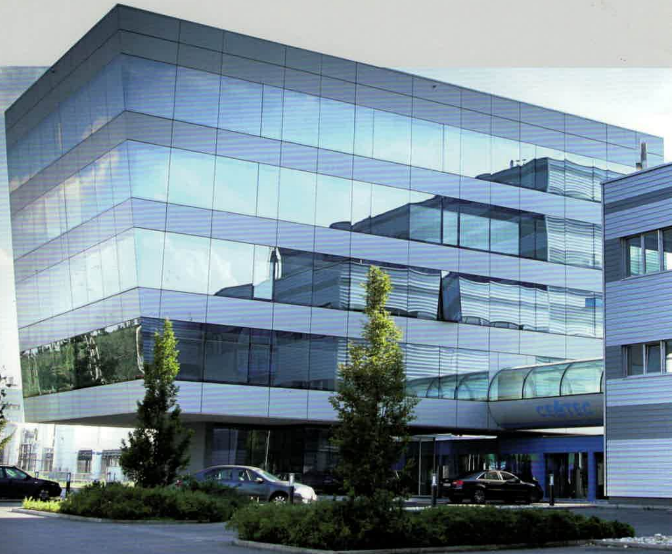
CEMTEC HEADQUARTERS IN ENNS AUSTRIA
