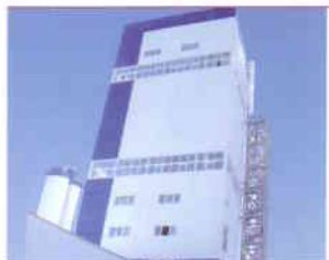
Production of Building materials
